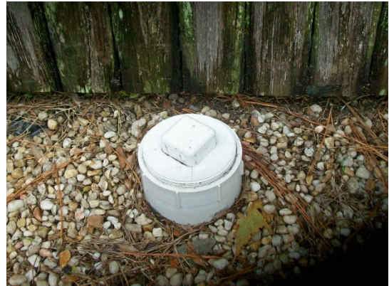
Undamaged Cleanout Cap & Assembly
